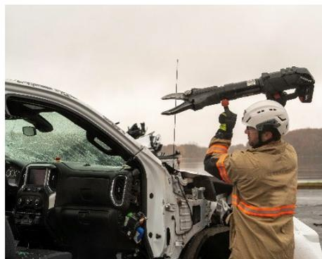
Figure 3. A responder operates a Holmatro Pentheon PCU50 Cutter, using the 360 rear handle for leverage (left). Another responder lifts a Genesis C236-SL3 EForce Cutter into place (right); note the length and back end design of the tool.
