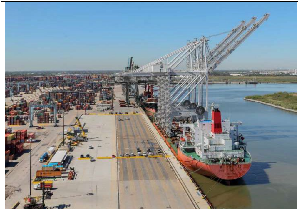
Figure 3. Heavy load carrier ZHEN HUA 13 delivers ZPMC cranes to a port terminal in Houston, TX. 16
