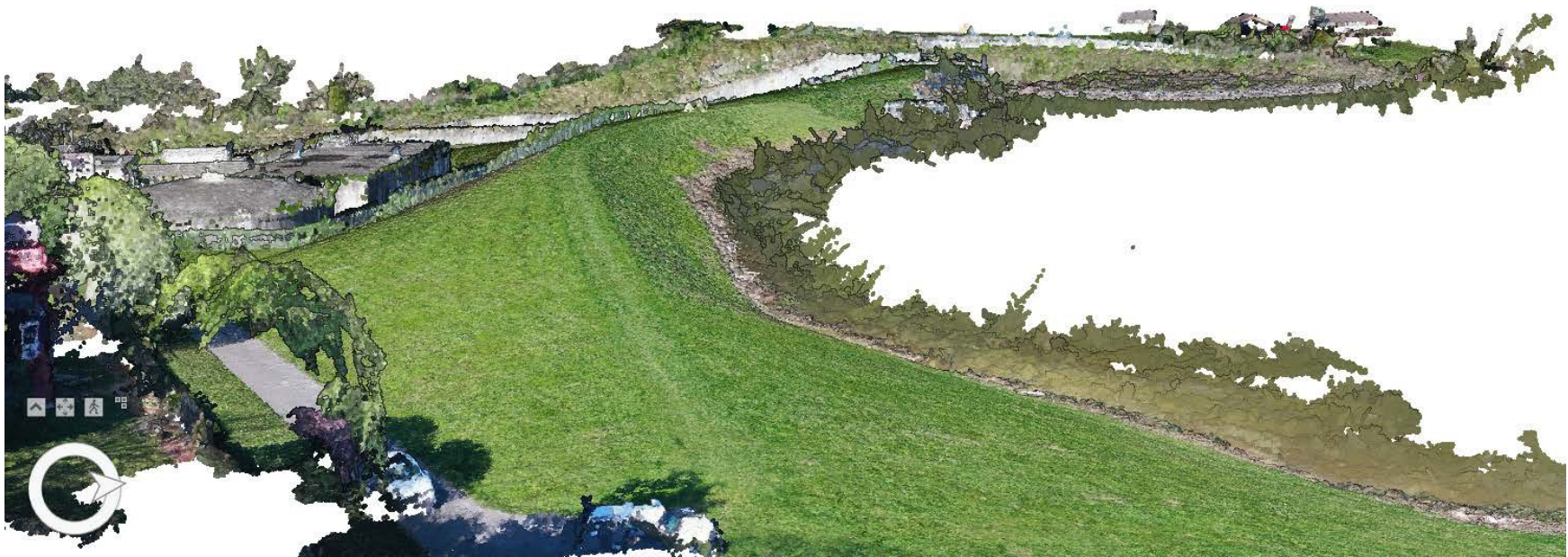
Representation of LIDAR data colorized from imagery from drone flight of Guist Creek Dam
