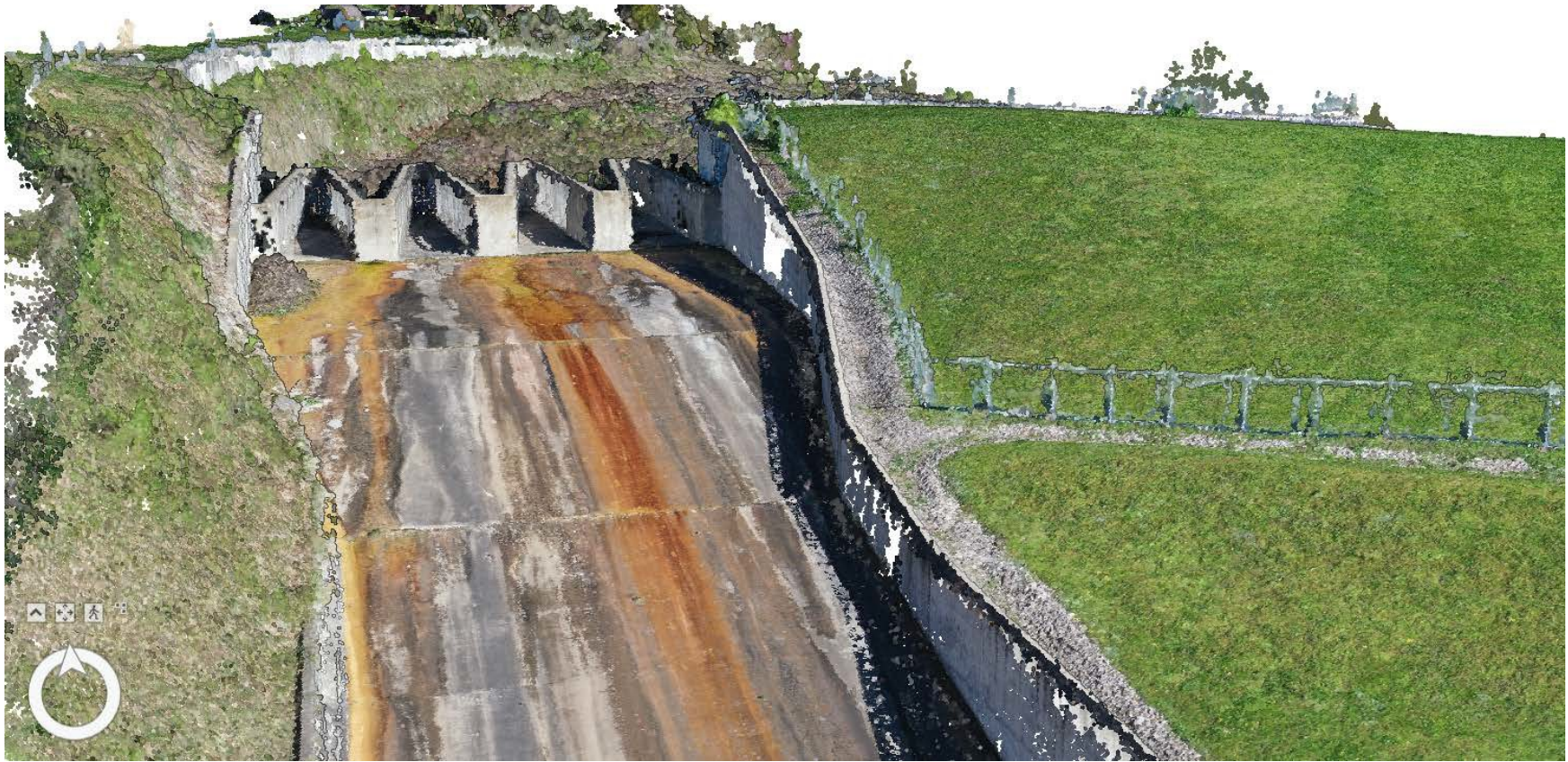
Representation of LIDAR data colorized from imagery from drone flight of Guist Creek Dam
