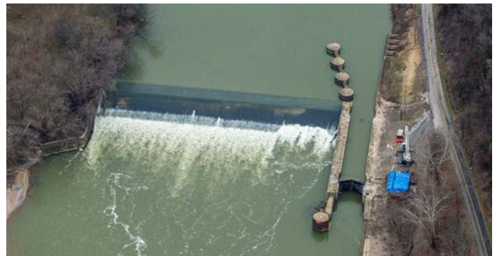
Most critical infrastructure is at risk from flooding. High risks may be present, but may be unknown or rapidly develop.
