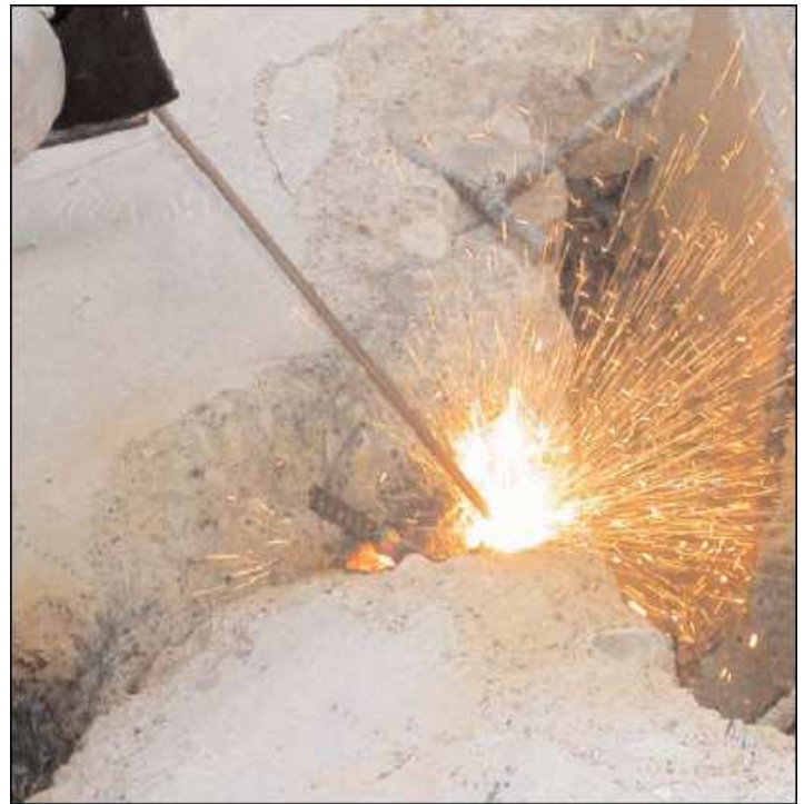
Figure 2. Exothermic cutting torch on rubble.
