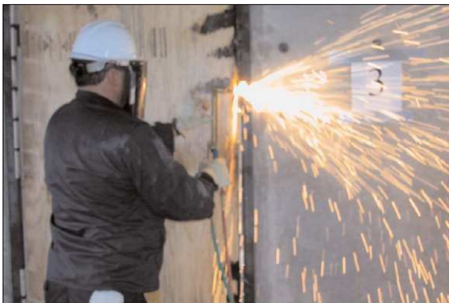
Figure 1. Tactical door entry with oxygen-acetylene torch.
