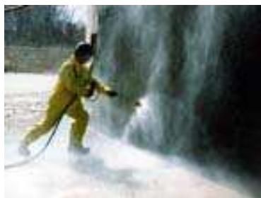
Figure 3. Pressure Washing
