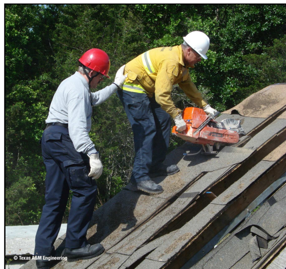
Figure 2. An emergency responder SME cuts composite wood roofing.
