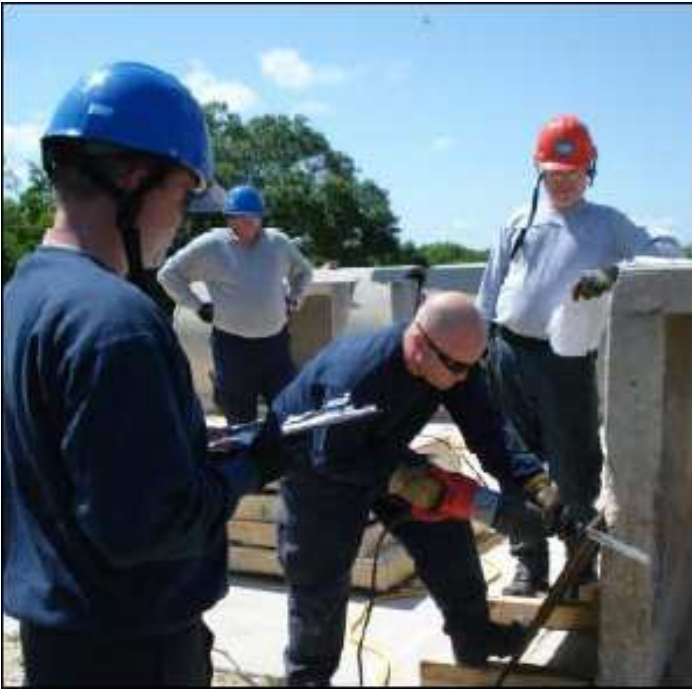
Figure 1. SMEs cut 1/2-inch plate steel using multipurpose reciprocating saw blades.
