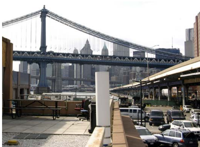
REMS sensor installation in New York City
