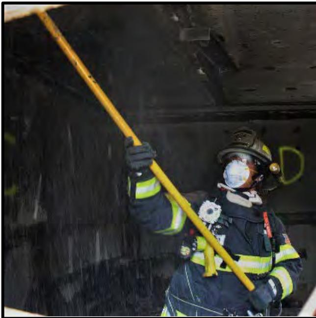
Figure 2-5 Ceiling Breach and Pull
