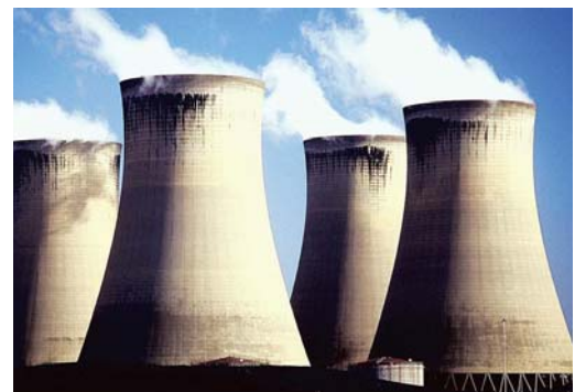
Nuclear Power Plant Cooling Towers
