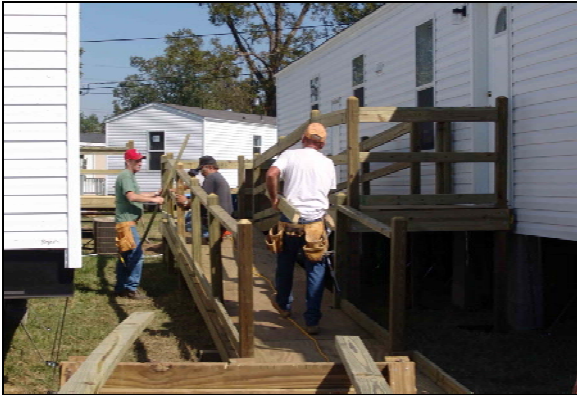
Figure 3. Workers build a ramp to create a wheelchair accessible manufactured home.
