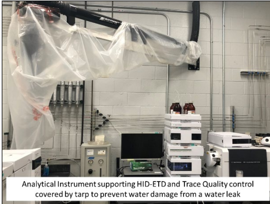
Figure 2-3. Laboratories also are experiencing roof leaks, sometimes directly above expensive equipment.
